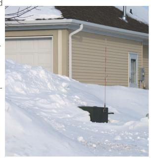
businesses in your area. The National Electric Code states to allow at least 10 feet in front of power equipment and 3 feet on the sides and back for line workers to be able to access the area in the event of an emergency.
