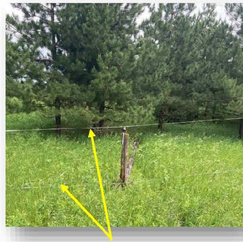
Lines still suspended even with pole broken and on ground (retrieved from Lake Region's Facebook)
