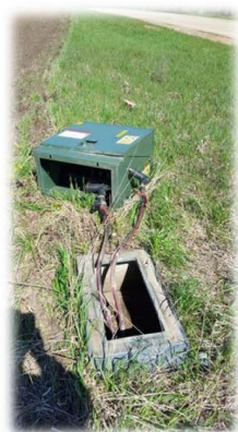
Operator of field cultivator knocked it off the base
