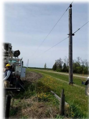
Operator of equipment hit pole, snapping it in half but lines remained in the air
